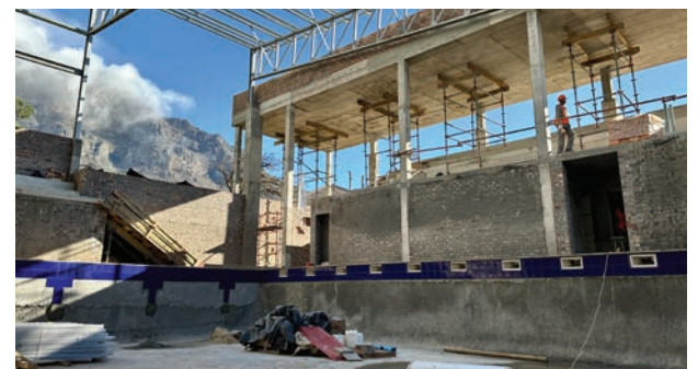
Aquatics Centre under construction will have a view of Table Mountain
