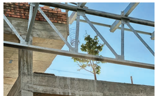
African Olive tree placed on the roof of the new complex in the ceremony
