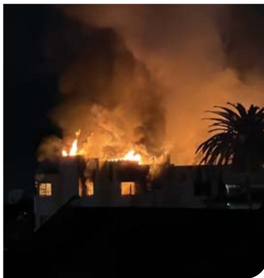
Apartment block fire
